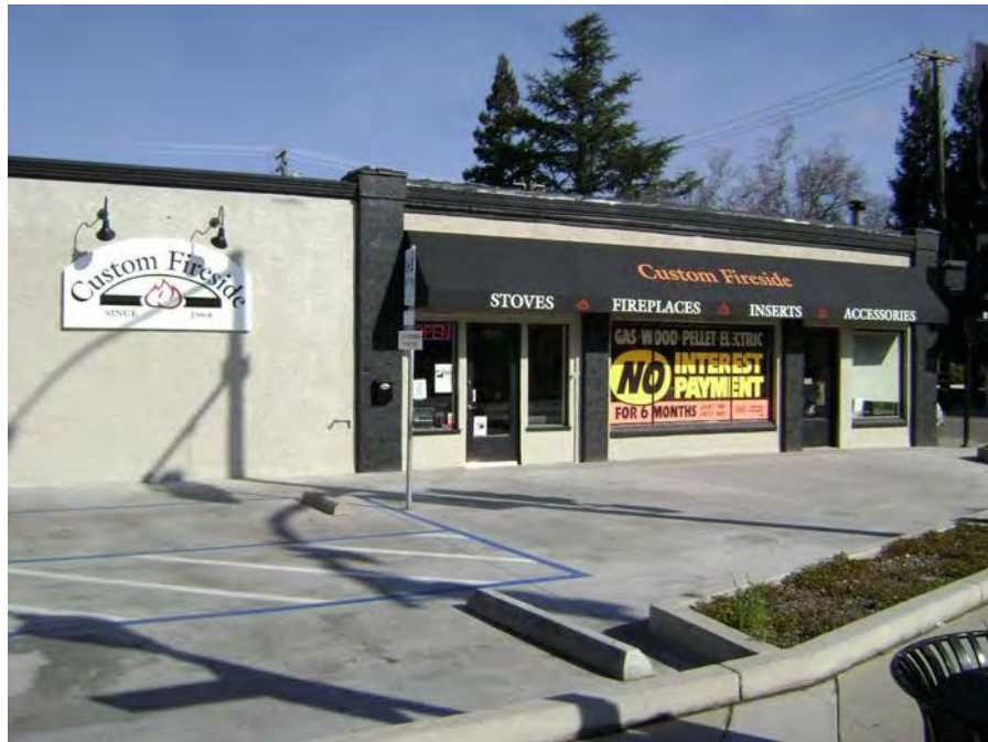
View of south (primary) façade (Page & Turnbull, 02/13/2012).
