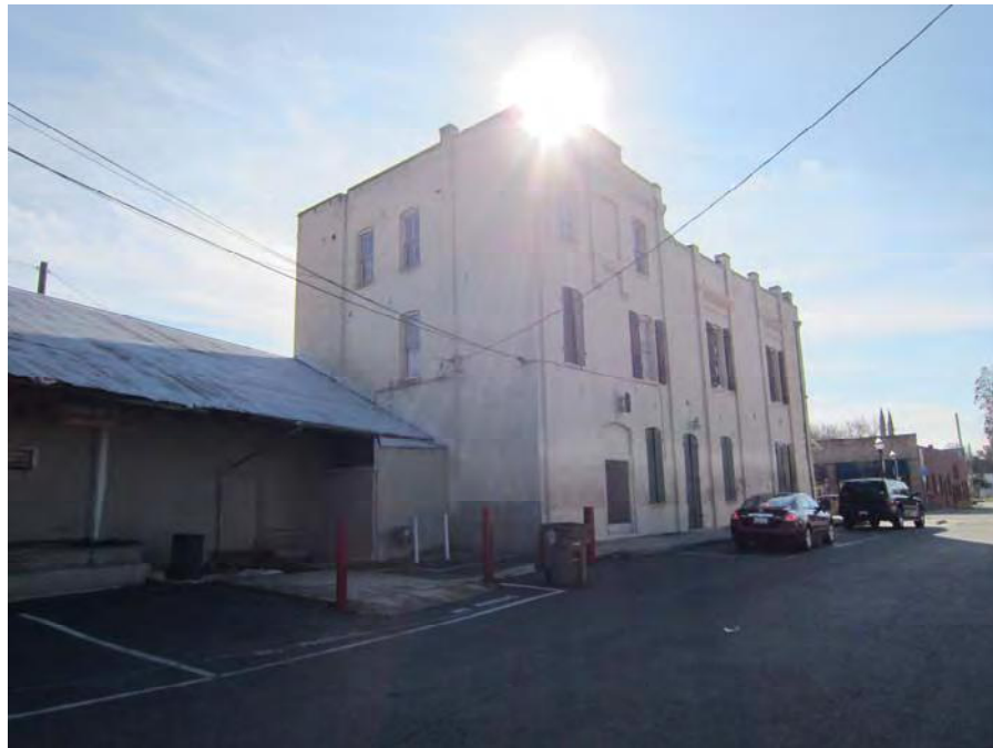
View of north and west facades of IOOF Building and adjoining warehouse building (Page & Turnbull, 02/13/2012).
