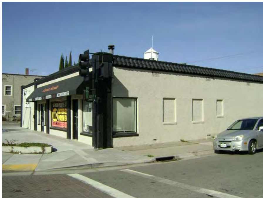
View of south (primary) and east (School Street) façades (Page & Turnbull, 02/13/2012).
