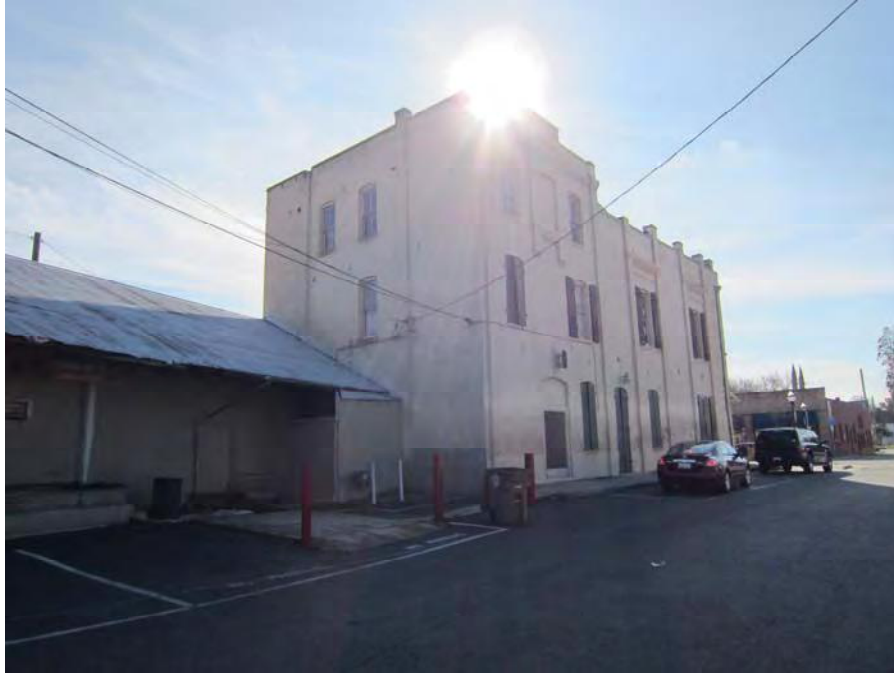
View of north and west facades of IOOF Building and neighboring warehouse building (Page & Turnbull, 02/13/2012).
