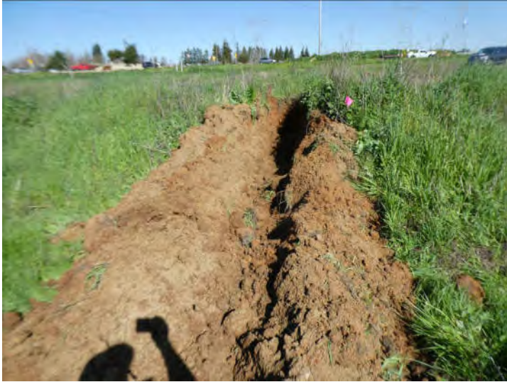
Photo #7: Northeastern soil piles Trench T-5
