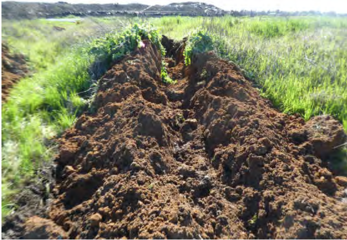
Photo #13: Northeastern soil piles Trench T-10
