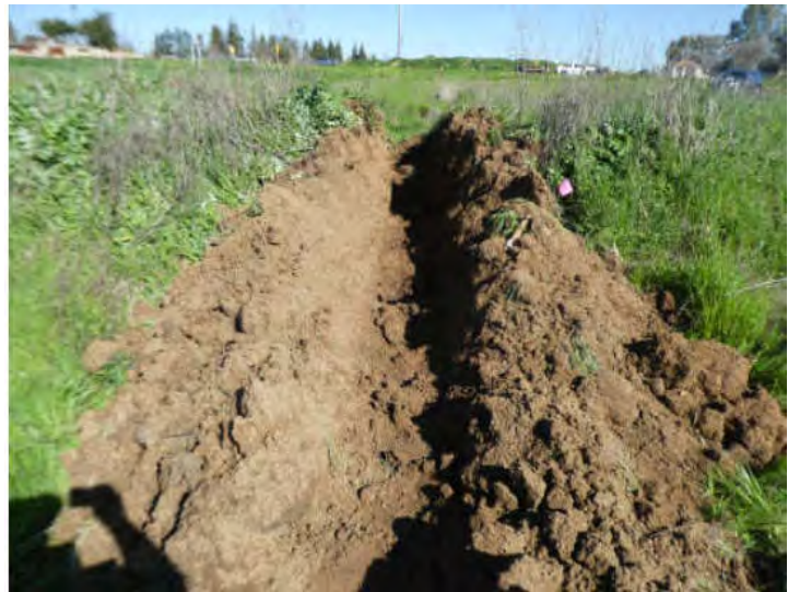
Photo #8: Northeastern soil piles Trench T-6
