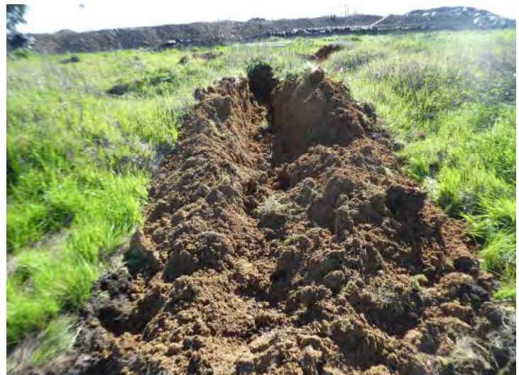
Photo #14: Northeastern soil piles Trench T-11
