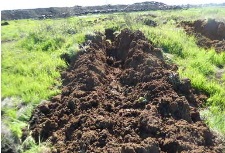
Photo #15: Northeastern soil piles Trench T-12
