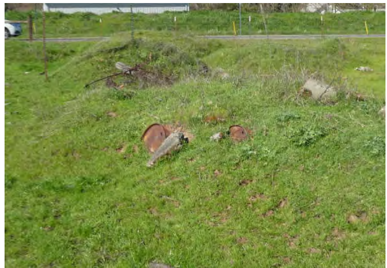
Photo #26: Western soil piles Trench T-9 - Concrete, metal debris (pre-trenching)
