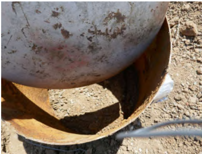
Photo #18: Anomalous features at southeast side of dwellings
