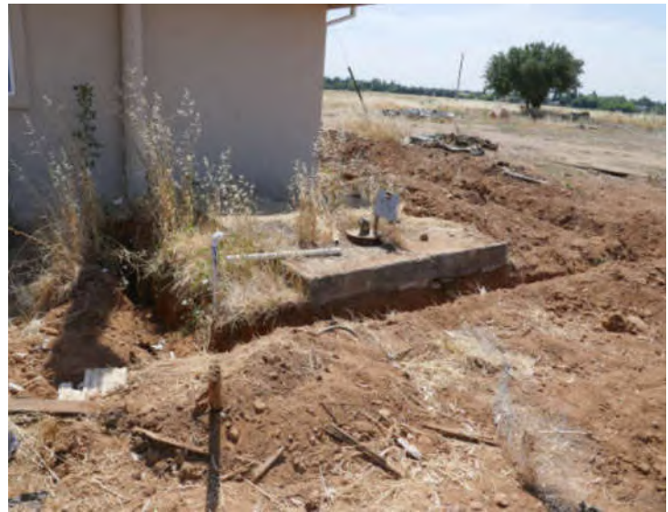
Photo #11: On-site water well at southwest corner of dwelling
