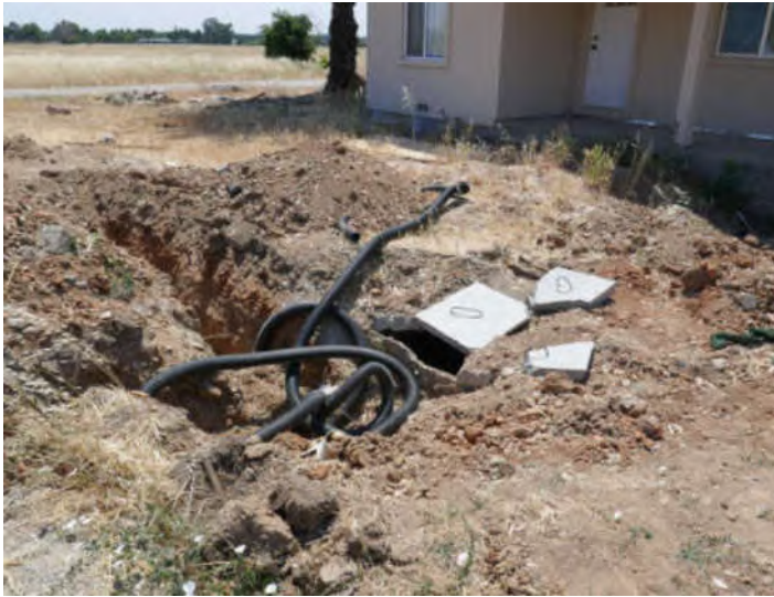
Photo #13: Septic vault on north side of dwelling
