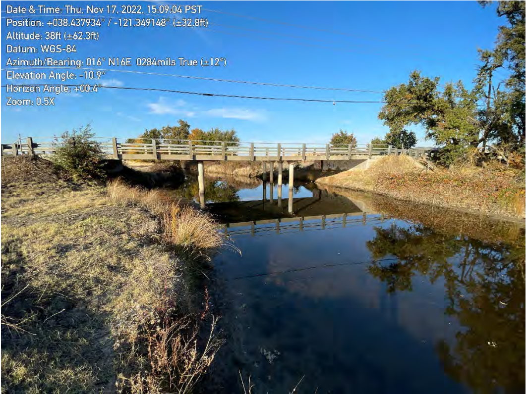
Photograph 7. Facing north (upstream) at the Sheldon Road bridge over Laguna Creek
