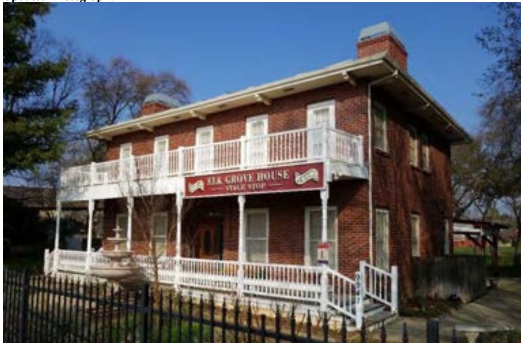
Photograph 1. View north of southwest and southeast elevations.
