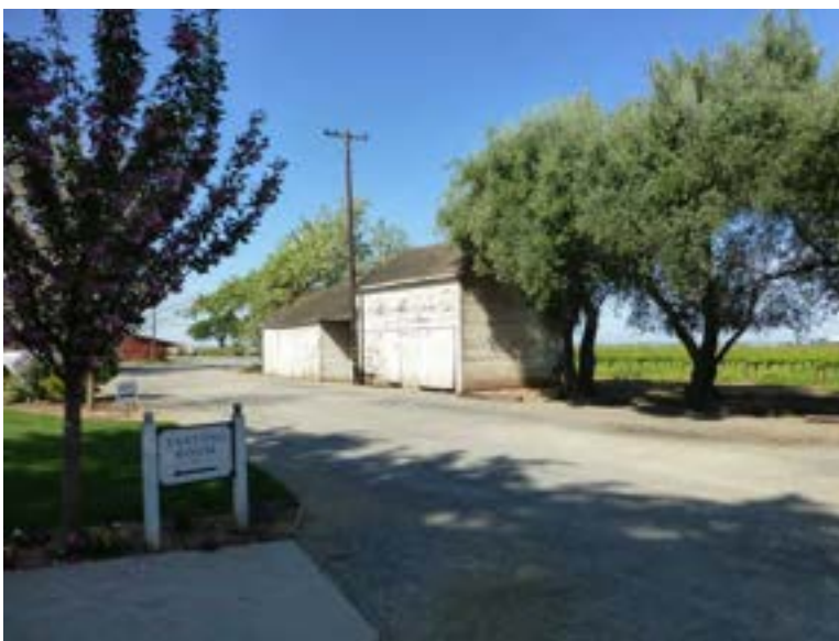
Photograph 3. View northwest of ancillary building. Taken 4/9/14, #0533.
