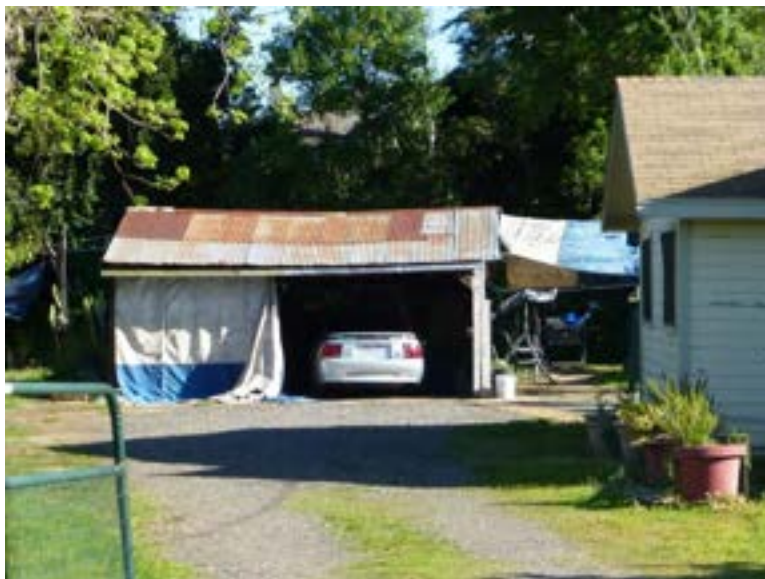
Photograph 2. View northwest of detached garage. Taken 4/10/14.
