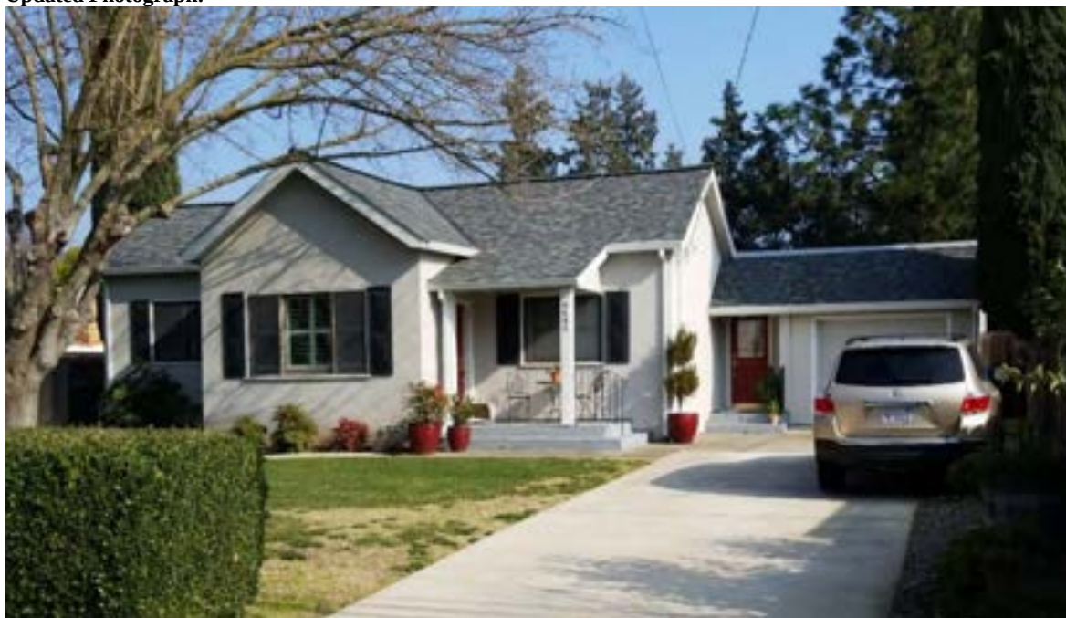
Photograph 1. View northeast of the west elevation.
