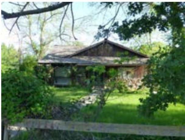
Photograph 5. South elevation of Residence 1. Camera facing north.
