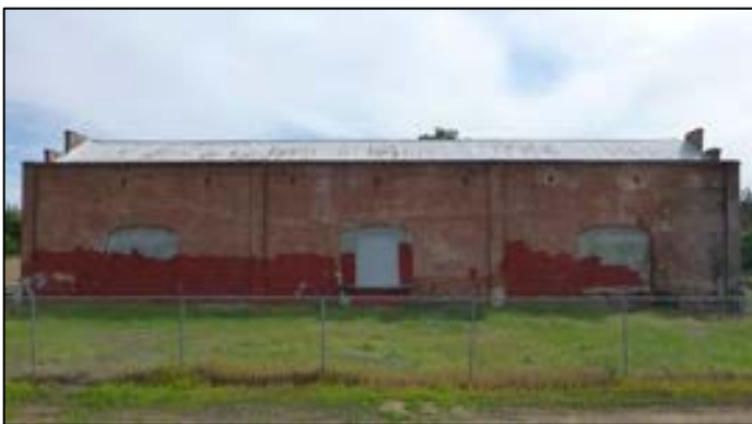
Photograph 15. West elevation of Bldg. 2. Camera facing east.
