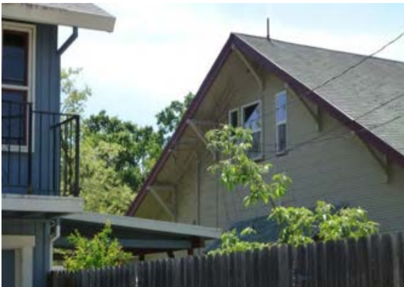
Photograph 2. View southwest of east elevation. Taken 4/9/14, #0561.
