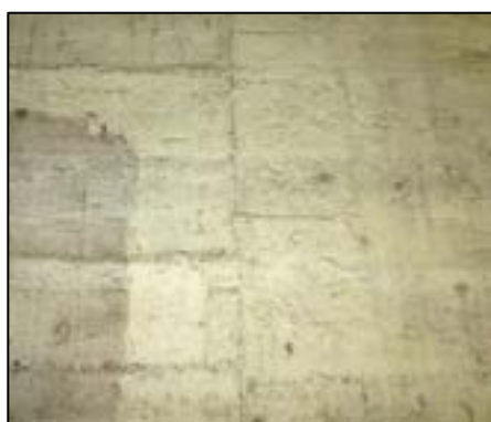
Photograph 11. Board-formed, reinforced concrete interior wall of Bldg. 5.
