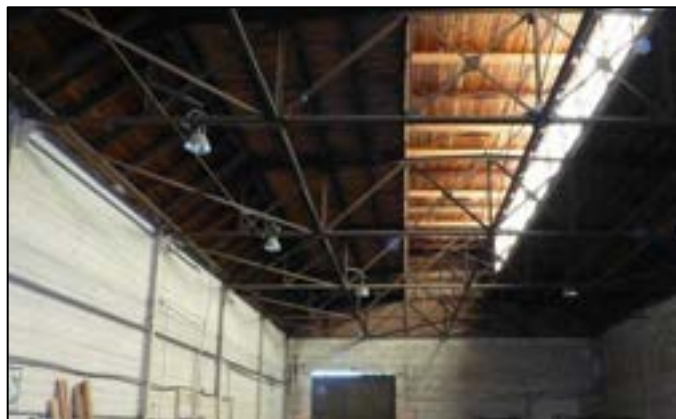
Photograph 10. Bldg. 6, by contrast, displays a steel-truss roof system and no interior posts due to the narrower width of the building.
