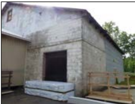
Photograph 17. Bldg. 4-north & west elevations of winery warehouse.
