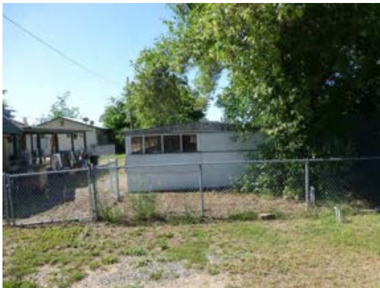
Photograph 2. View southeast of Buildings 1 and 3. Taken 5/11/14.
