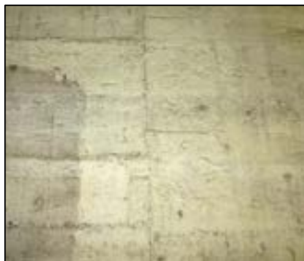
Photograph 11. Board-formed, reinforced concrete interior wall of Bldg. 5.
