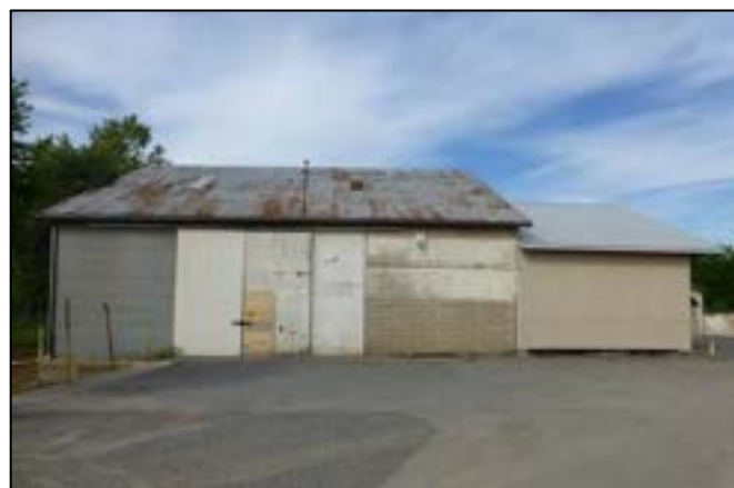
Photograph 14. East elevation of Bldg. 4. Less than half of the building displays its original concrete-block walls. The southern half of the building was rebuilt corrugated metal in 1984
