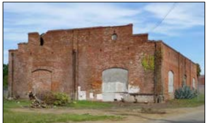
Photograph 3. South and east elevations. Camera facing northwest.
