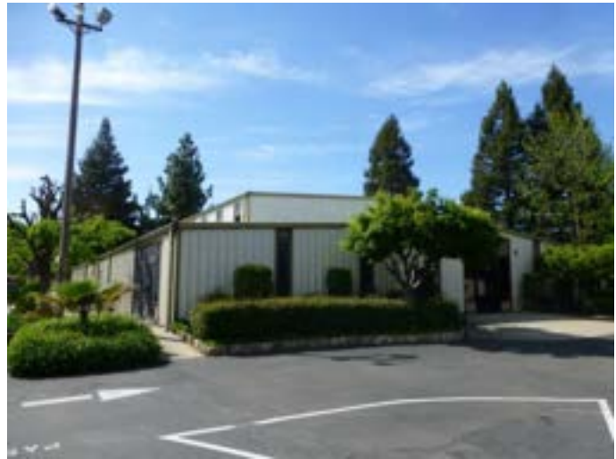
Photograph 5. View northwest of church offices.
