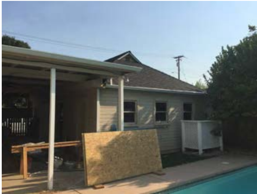
Photograph 6. View northeast of garage.
