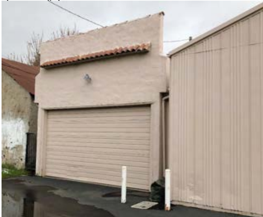
Photograph 1: View northwest of south elevation.
