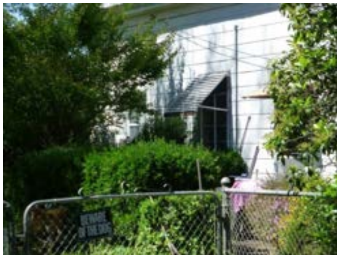
Photograph 2. View northwest of south elevation.
