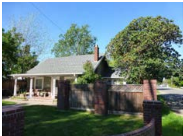
Photograph 2. View southwest of east elevation. Taken 4/10/14
