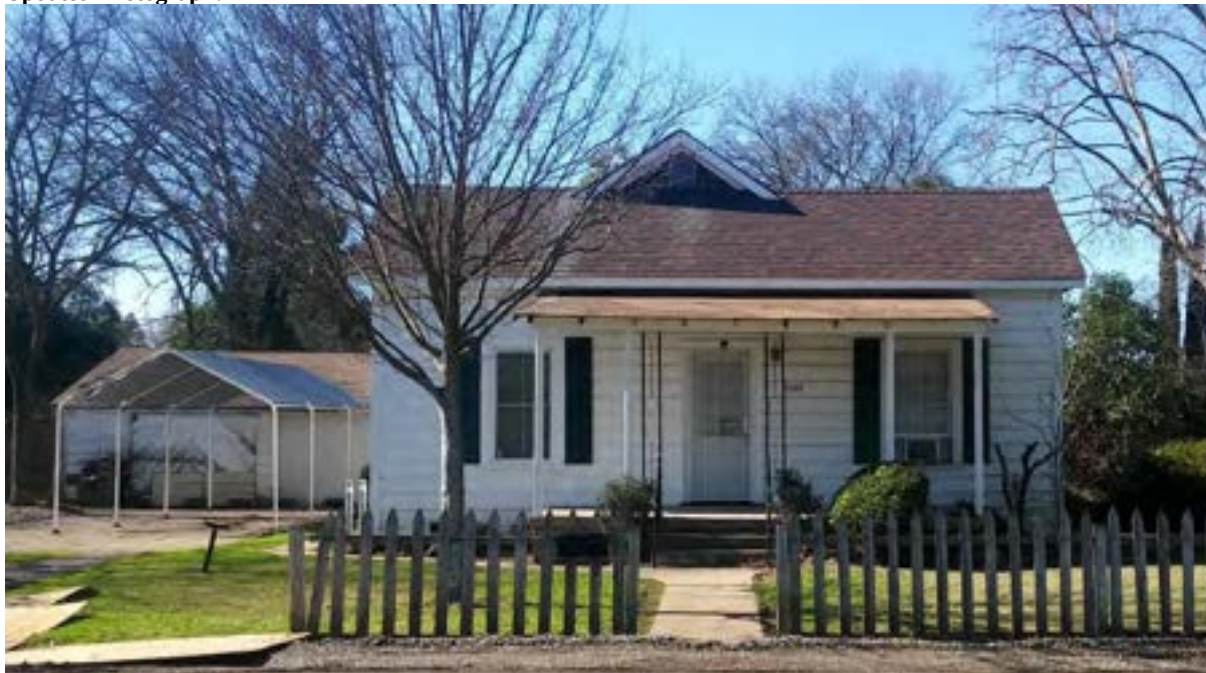
Photograph 1. View west of east facade.
