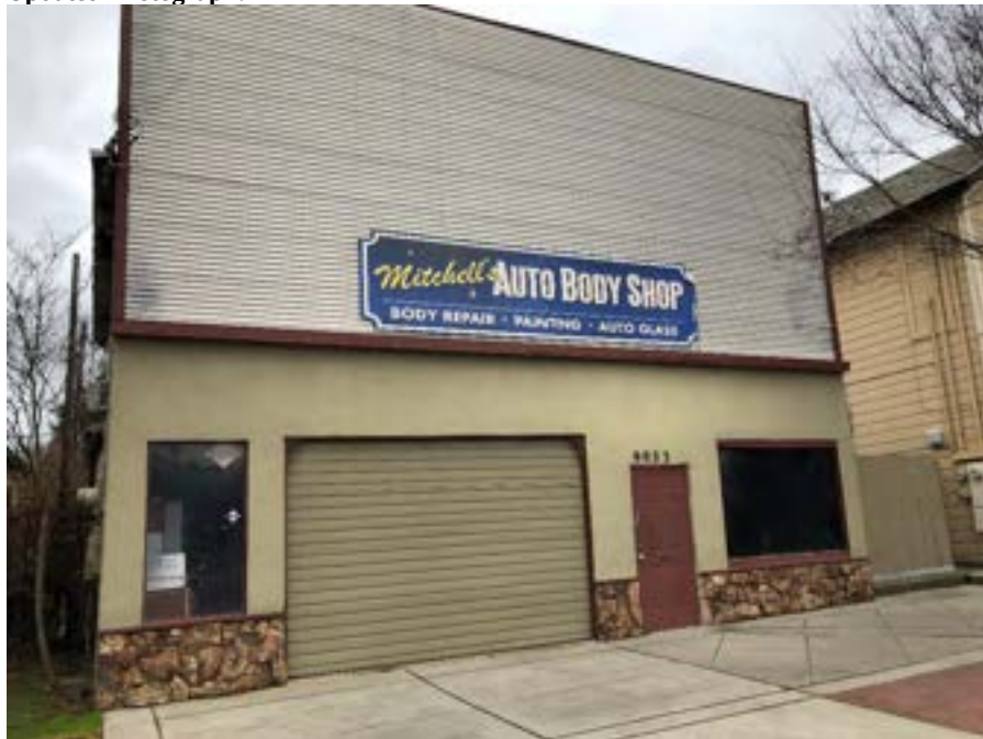
Photograph 1: View north of south elevation.
