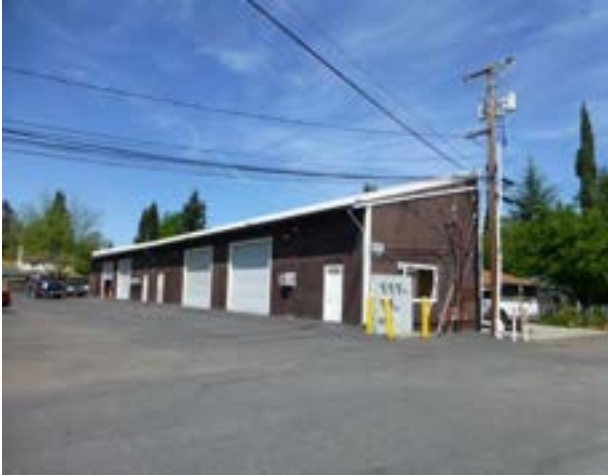
Photograph 3. Building C. View northeast. Taken 4/9/14.
