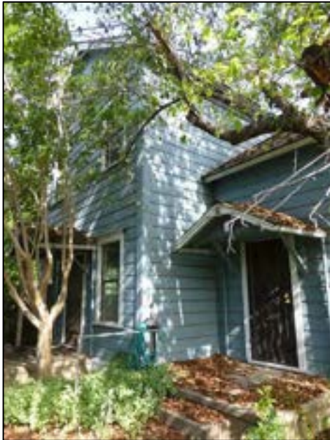
Photograph 3. Front (south) façade. Camera facing northwest.
