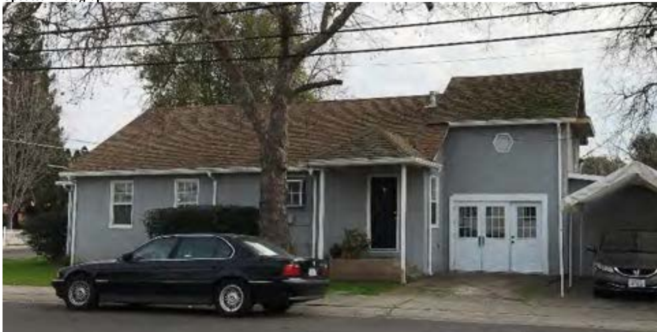
Photograph 1: View south of north elevation.
