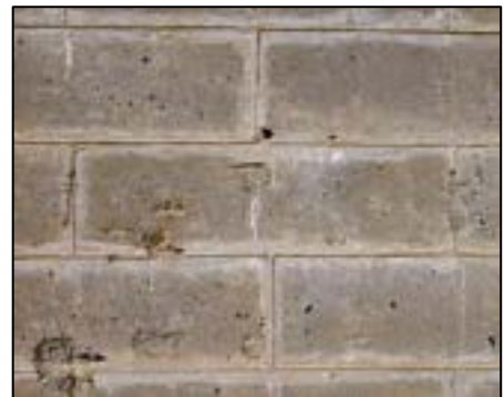
Photograph 19. Bldg. 4-Closeup of original concrete block wall.
