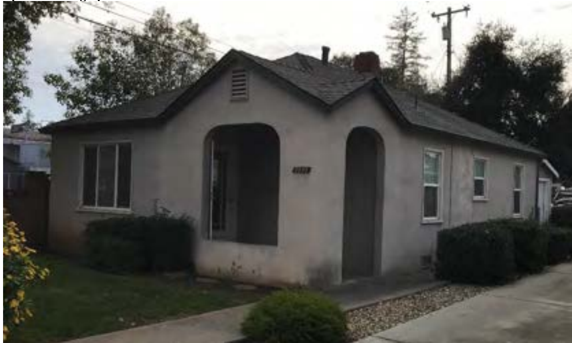
Photograph 1: View southwest of east and north elevations.
