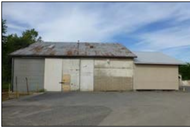
Photograph 12. East elevation of Bldg. 4. Less than half of the building displays its original concrete-block walls. The southern half of the building was rebuilt corrugated metal in 1984
