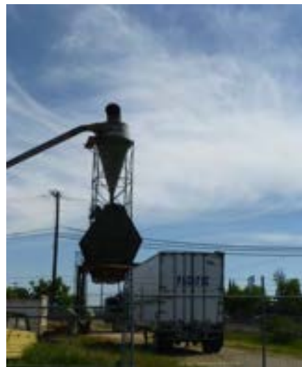
Photograph 6. Machinery. View south.
