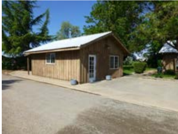
Photograph 3. View northwest of Office Building 2.
