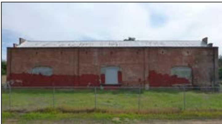
Photograph 2. West elevation. Camera facing east.
