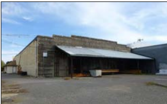
Photograph 3. South and west elevations of Bldg. 5. Note the unpainted, board-formed, reinforced concrete wall, a character-defining feature of this 1915 industrial building.
