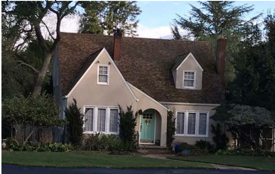
Photograph 1. View east of the west elevation.
