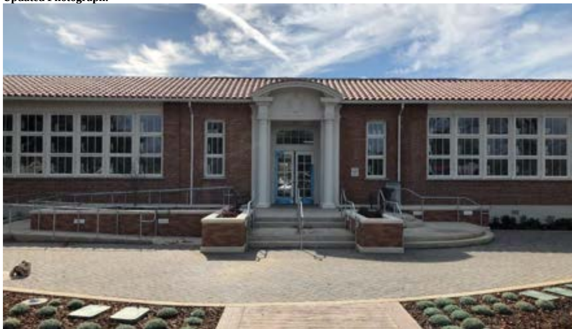
Photograph 1: View south of north elevation.
