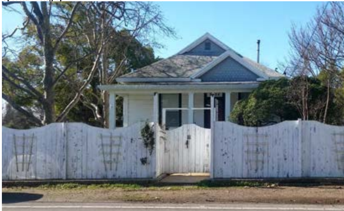
Photograph 1. View west of east façade.
