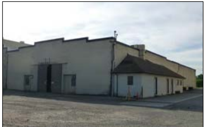
Photograph 2. North and west elevations of Bldg. 5. The half-hipped, truck-scale office appended to the west elevation is not an original feature of the building as constructed in 1915.
