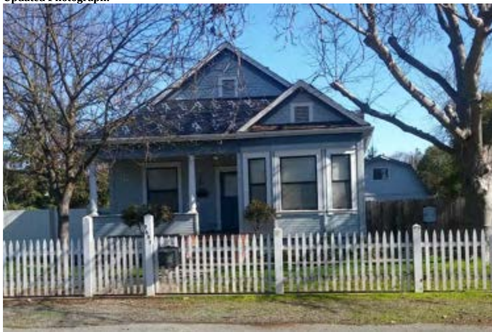
Photograph 1. View east of west façade.
