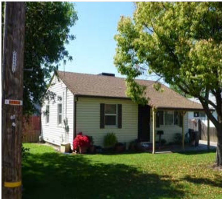
Photograph 2. View southwest of north and east elevations.
