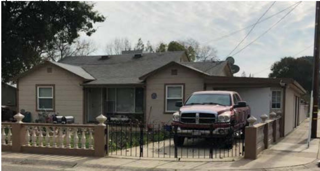
Photograph 1. View southeast of the north elevation.
