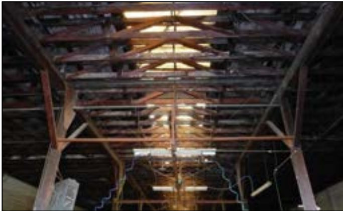
Photograph 9. Bldg. 5. features a timbered -truss roof system supported by knee-braced, square timber posts.
