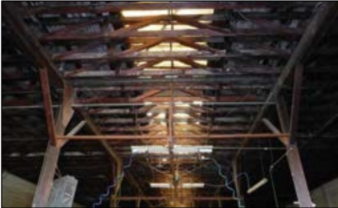
Photograph 5. Bldg. 5. features a timbered -truss roof system supported by knee-braced, square timber posts.
