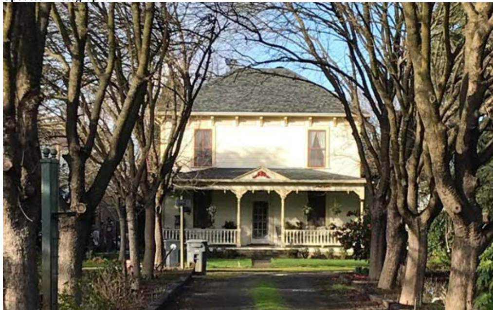
Photograph 1. View north of south elevation.
