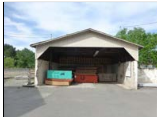
Photograph 10. East elevation of non-contributing storage bldg.
