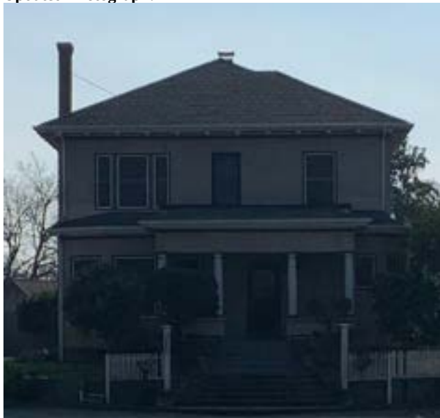
Photograph 1. View southwest of the east elevation.
