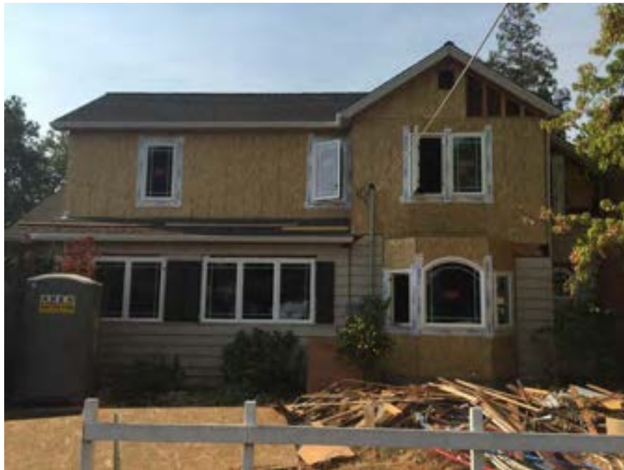
Photograph 3. View south of north elevation depicting large room addition, second-story addition, and new windows.
