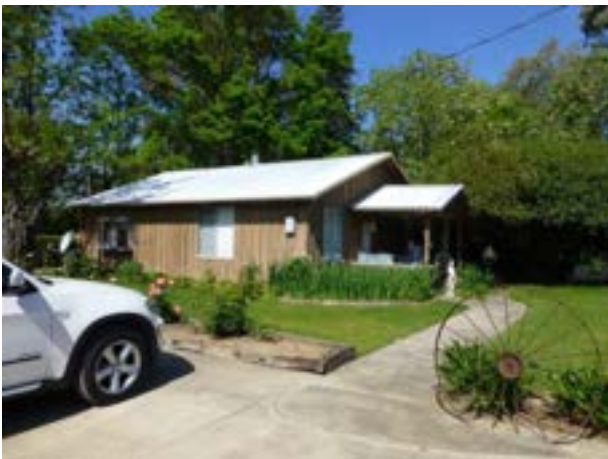
Photograph 4. View northwest of Office Building 1.
