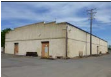
Figure 10. Bldg. 3- Fermenting & Wine Storage Facility.
