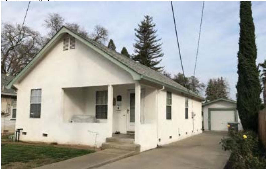
Photograph 1: View northeast of west and south elevations.
