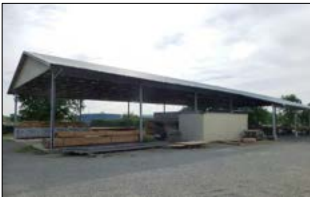
Photograph 9. West & north elevation of non-contributing pole barn.
