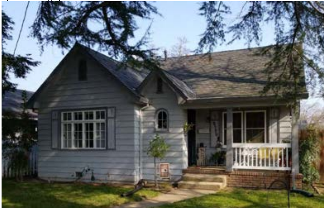
Photograph 1. View northeast of west elevation.
