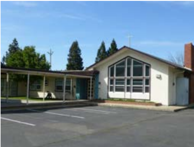
Photograph 4. View northwest of education building.
