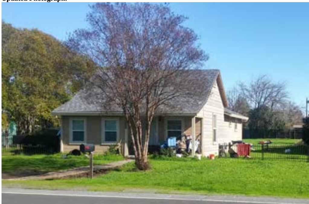
Photograph 1. View northeast of west and south elevations.
