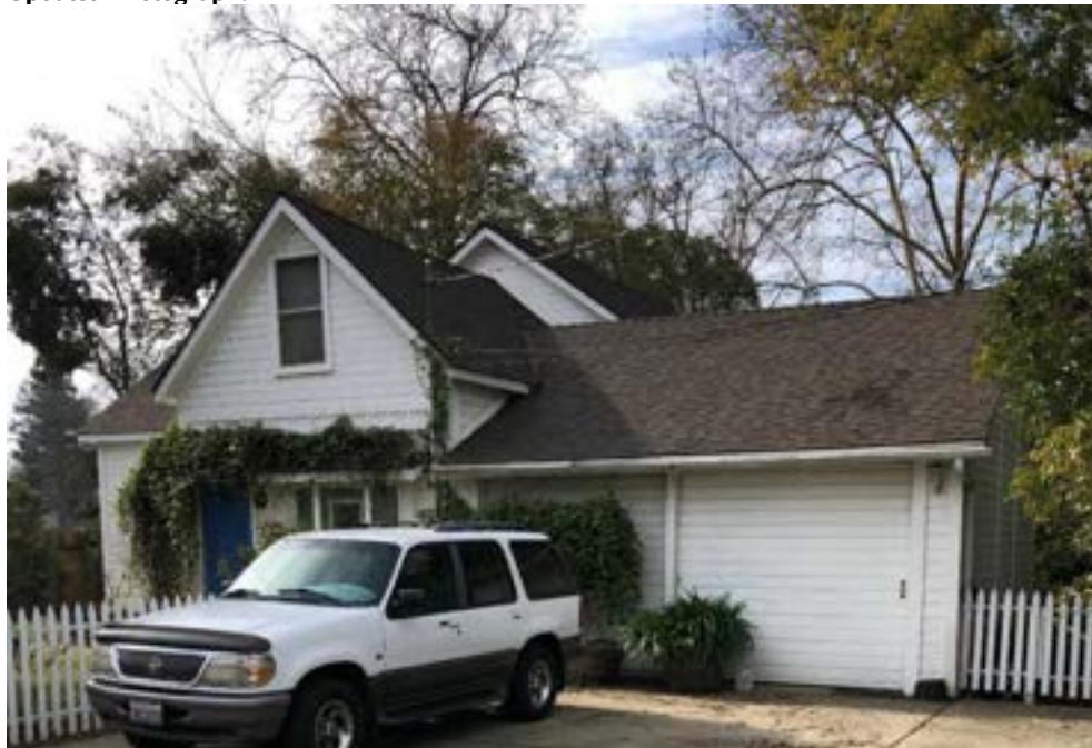
Photograph 1. View southwest of the east elevation.
