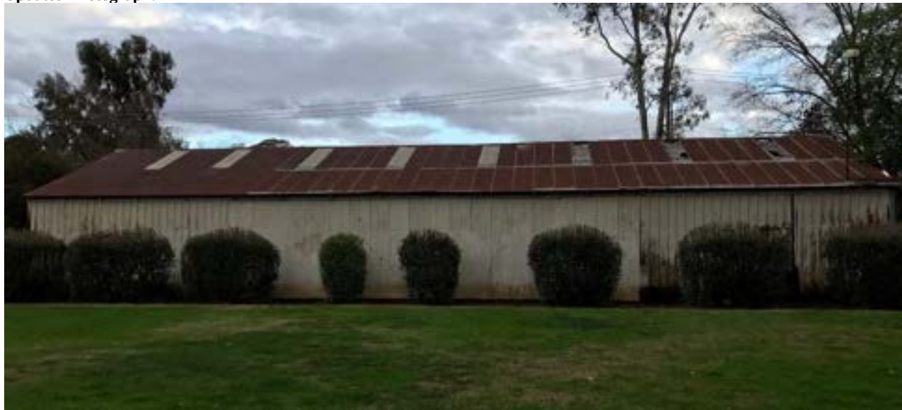
Photograph 1. View east of the west elevation.
