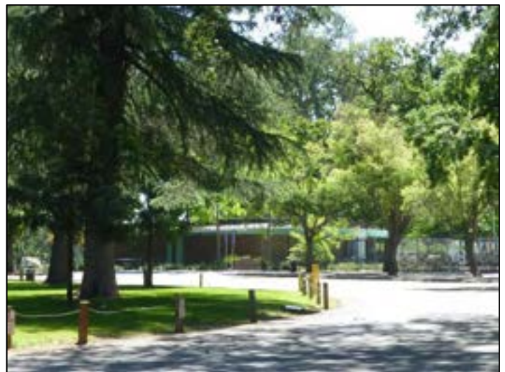
Photograph 11. View southeast of the swim center.
