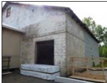
Figure 11. Bldg. 4-Winery Warehouse.
