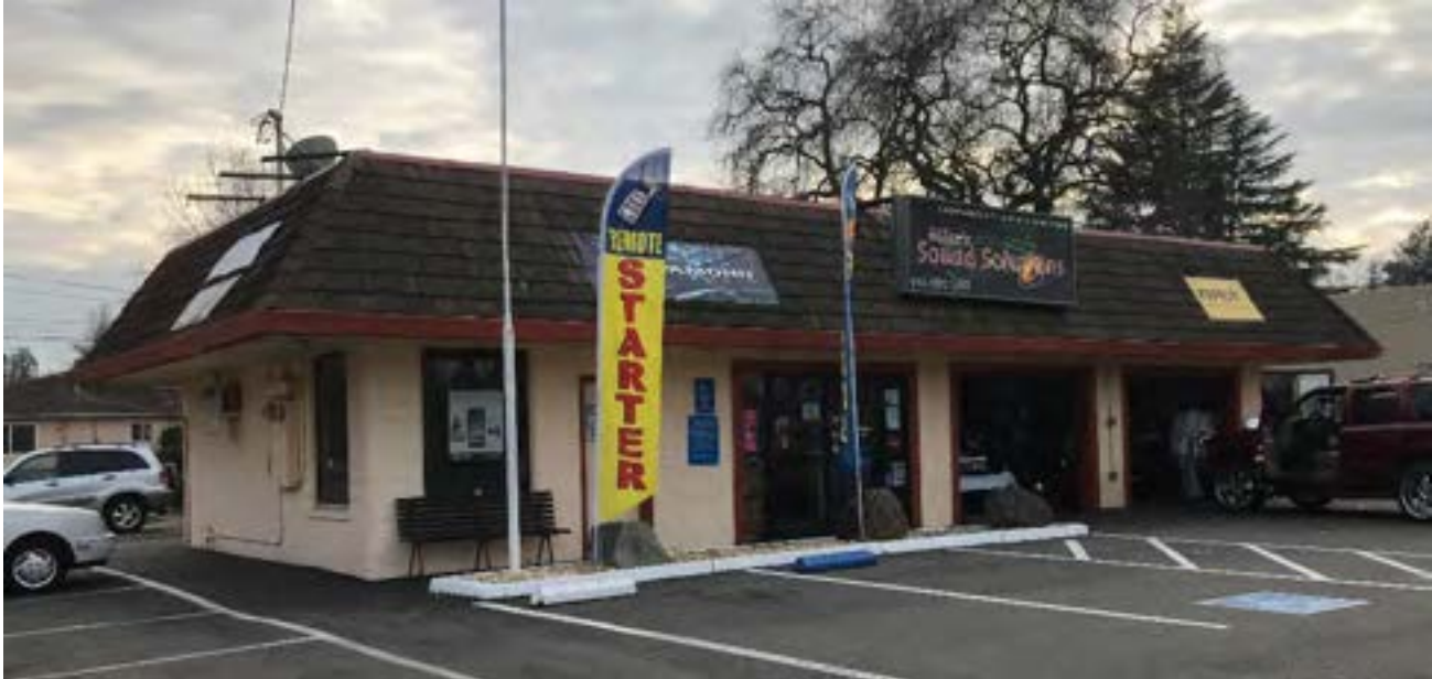
Photograph 1: View southwest of east and north elevations.
