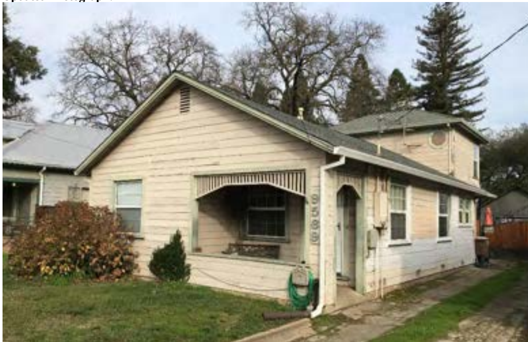
Photograph 1: View northeast of west and south elevations.
