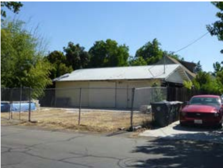
Photograph 3. View northeast of workshop. Taken 5/11/14, # 0019.
