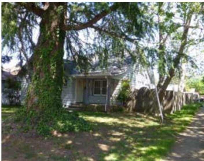
Photograph 2. View northeast of south and west elevations.
