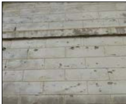
Photograph 18. Bldg. 4-Section of concrete-block wall.
