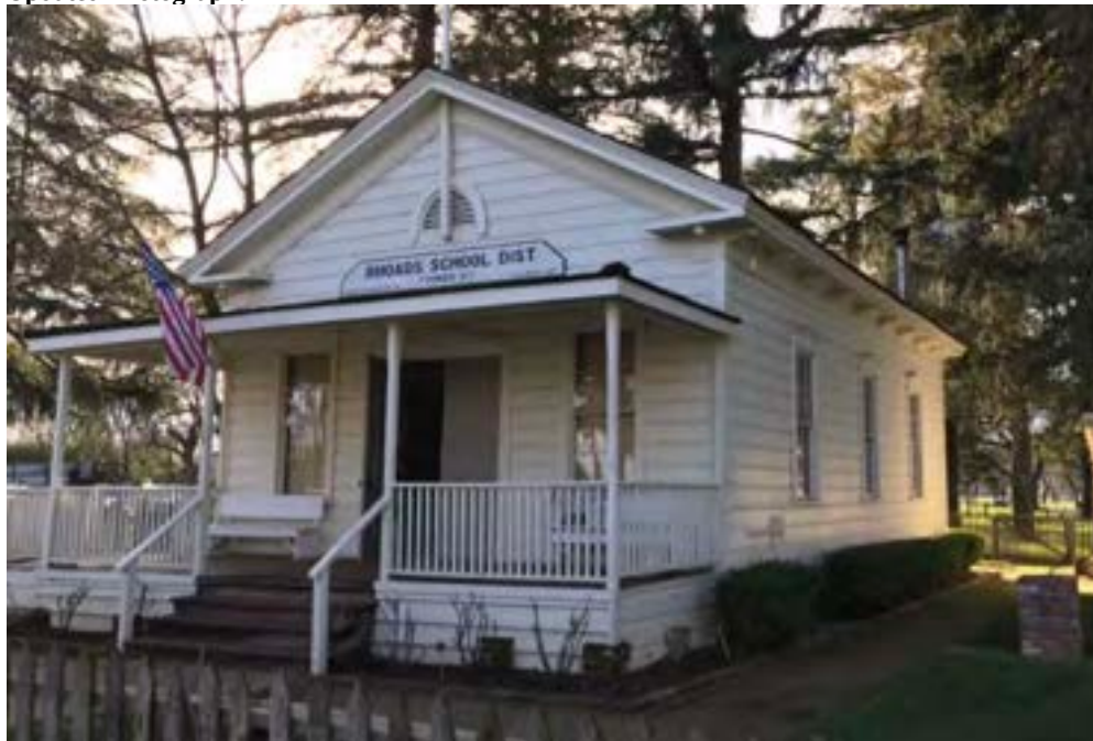
Photograph 1. View north of east and north elevations.
