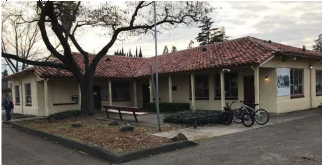
Photograph 1: View southwest of east and north elevations.
