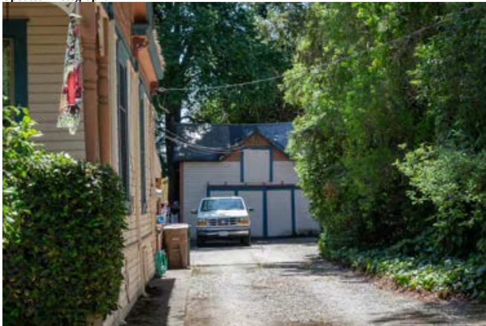
Photograph 1. View south of the north elevation.
