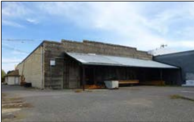
Photograph 4. South and west elevations of Bldg. 5. Note the unpainted, board-formed, reinforced concrete wall, a character-defining feature of this 1915 industrial building.
