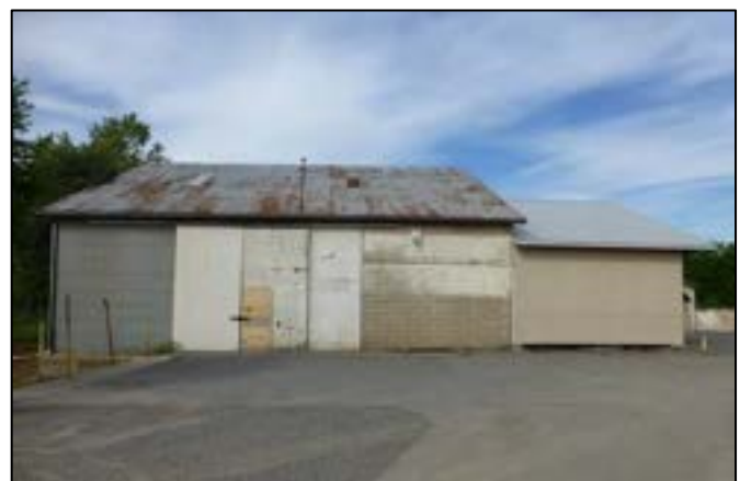
Photograph 14. East elevation of Bldg. 4. Less than half of the building displays its original concrete-block walls. The southern half of the building was rebuilt corrugated metal in 1984
