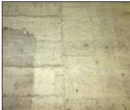
Photograph 7. Board-formed, reinforced concrete interior wall of Bldg. 5.
