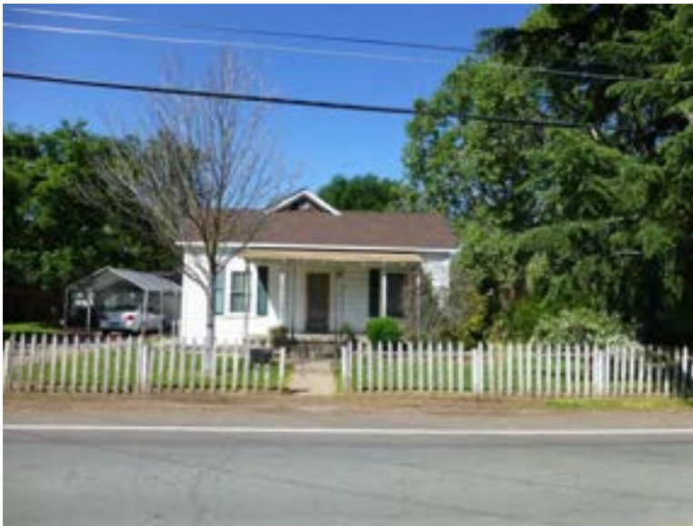
Photograph 3. View west of east façade. Taken 4/10/14, # 0644.
