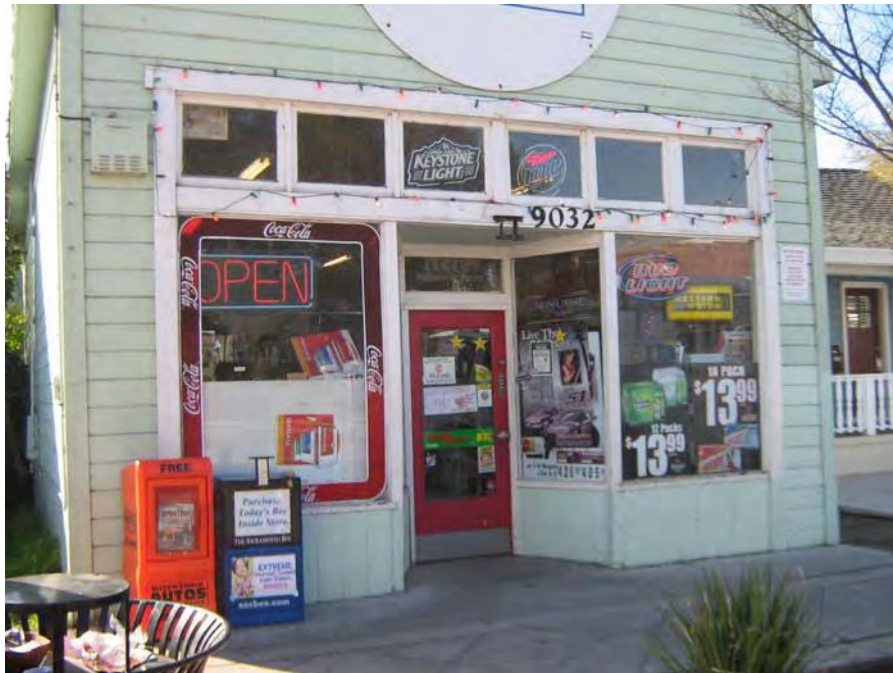
Detail view of north facade storefront (Page & Turnbull, 02/13/2012).
