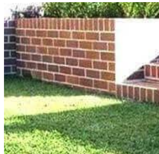
13 4 FT HIGH BRICK WALL - COLOR PER ELEVATIONS
