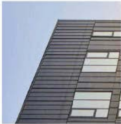
FIBER CEMENT PANEL (RANDOM BATTEN SIDING) (RBS): LIGHT OR DARK COLOR
