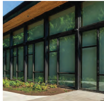
8 GLASS STOREFRONT WITH BRAKE METAL SYSTEM
