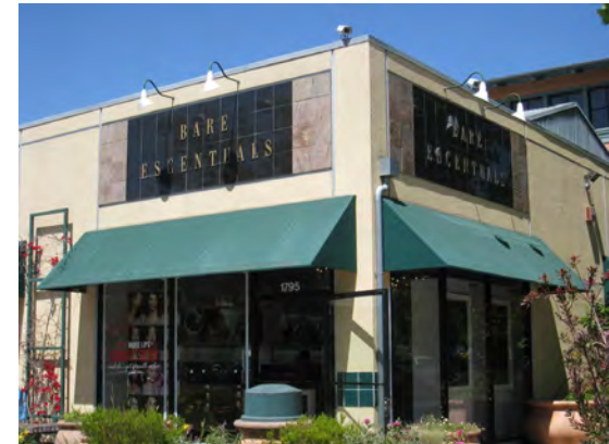
Glazing, lighting and awnings enhance facade
