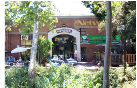
Building oriented to drainage channel
