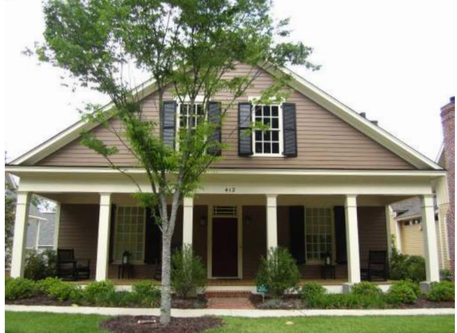
Detached Building Illustrative Photo
