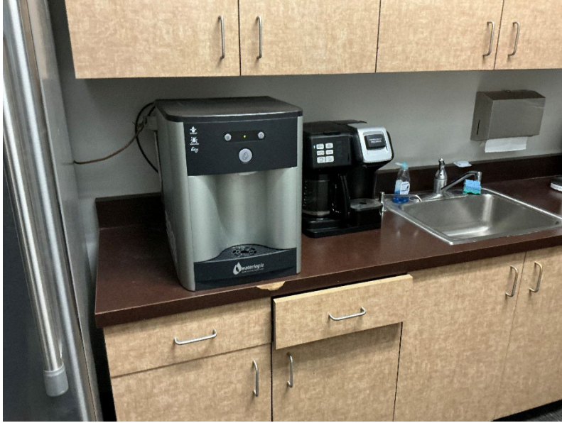
First floor Finance Area 18x14 Countertop hot/cold water dispenser (no drain access)
