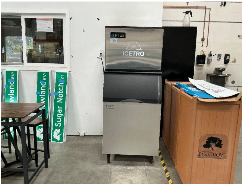
First Floor Warehouse 36x74 Bin Ice Machine with waterline off filter with drain
