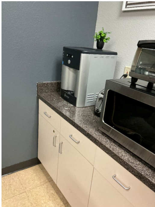
Second Floor – Breakroom 14x19 Countertop hot/cold water dispenser (no drain access)
