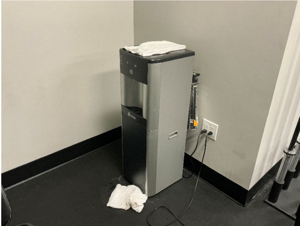
Fitness Room 14x41 Standalone hot/cold water dispenser (No drain access)
