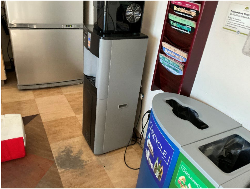
Breakroom 40x13 Standalone hot/cold water dispenser (no drain access)
