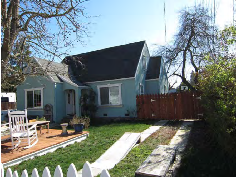
View of north and west façades (Page & Turnbull, 02/2012).
