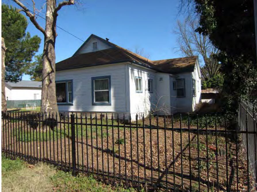
View of east (rear) and south façades (Page & Turnbull, 02/2012).
