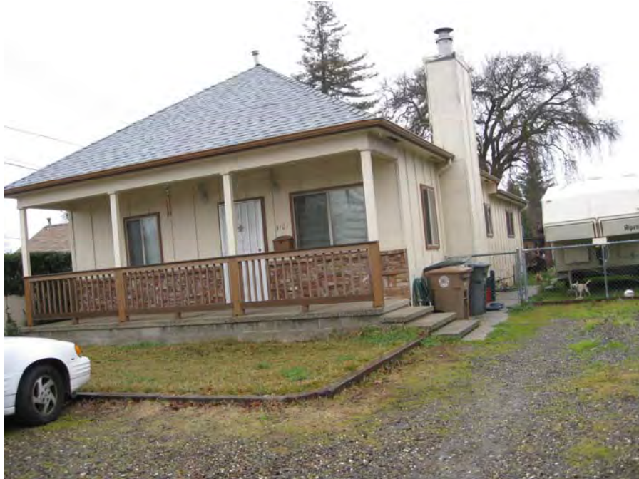
View of south and east facades (Page & Turnbull, 02/13/2012).
