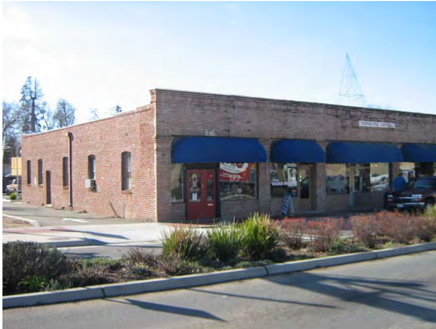
View of north and east facades (Page & Turnbull, 02/13/2012)
