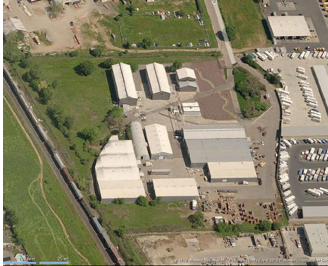
Gibson Winery, 9750 Kent Street. Photograph from Microsoft Corporation, 2012.
