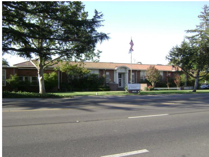
Administration Building, 8820 Elk Grove Boulevard. Photograph by Page & Turnbull, 2012.
