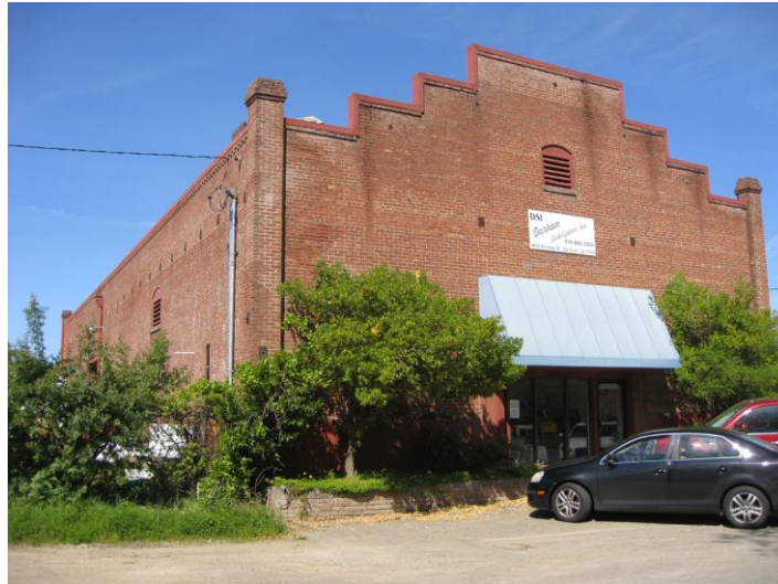
Da Roza and Neves Warehouse, 9678 Railroad Street, looking east. Photograph by Page & Turnbull, 2012.
