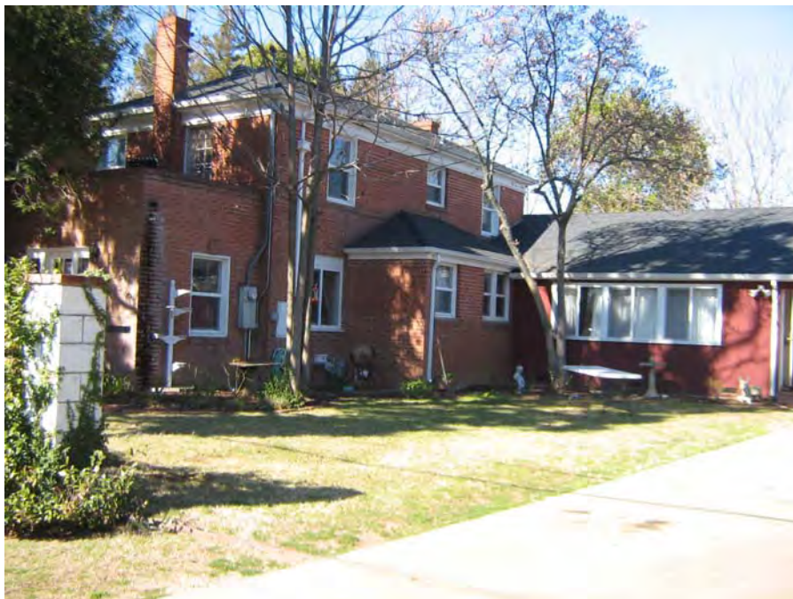
South and east facades with rear addition (Page & Turnbull, 02/15/2012).
