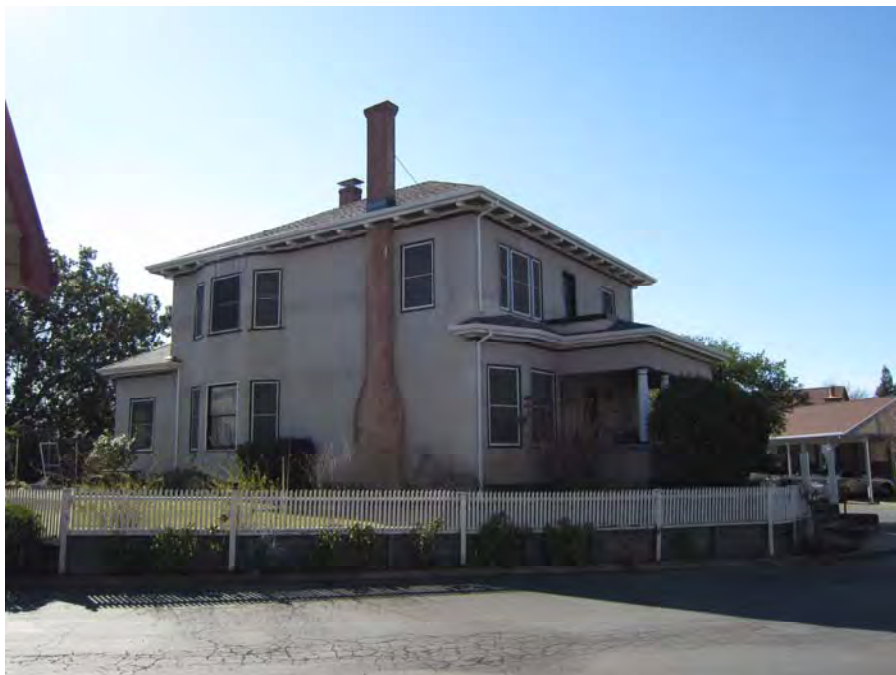
View of north and west facades (Page & Turnbull, 02/2012)
