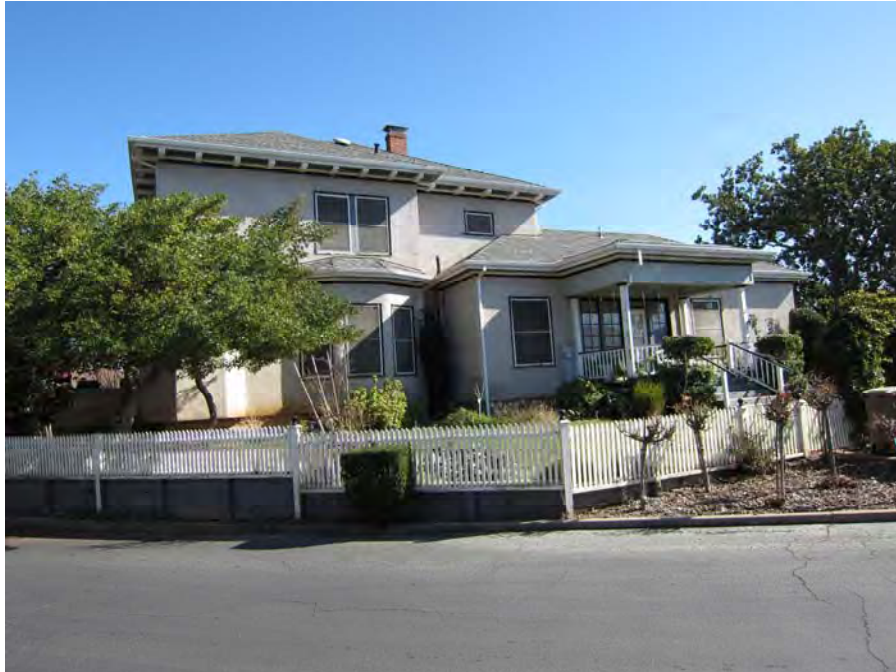
View of east façade (Page & Turnbull, 02/2012).
