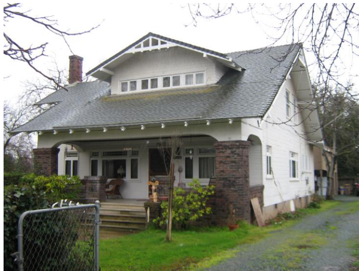
Haynes Residence, 9060 Grove Street, looking southwest. Photograph by Page & Turnbull, 2012.
