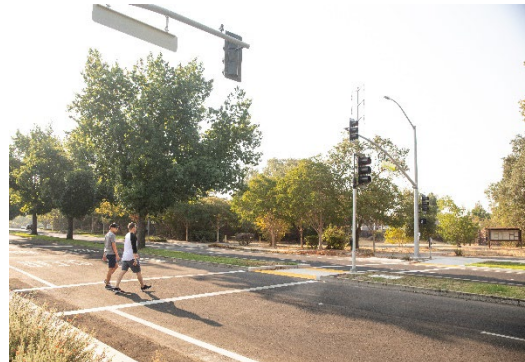
Figure 24. Signalized pedestrian crossing in Elk Grove
