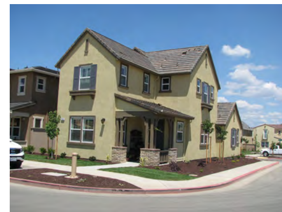
Architectural elements on all facades fronting public street
