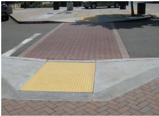
Ramp and warning strip
