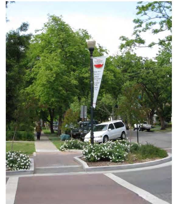
Bulbout at pedestrian crossing
