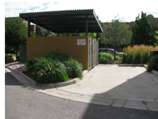
Paved and landscaped trash enclosure
