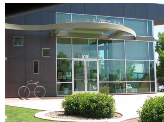
Entrance enhanced with decorative awning
