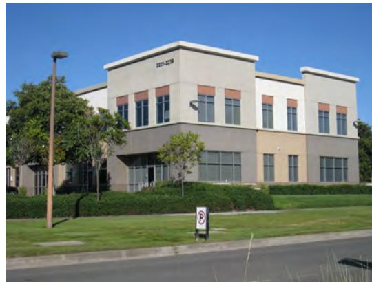
Consistent façade elements on multiple sides of building
