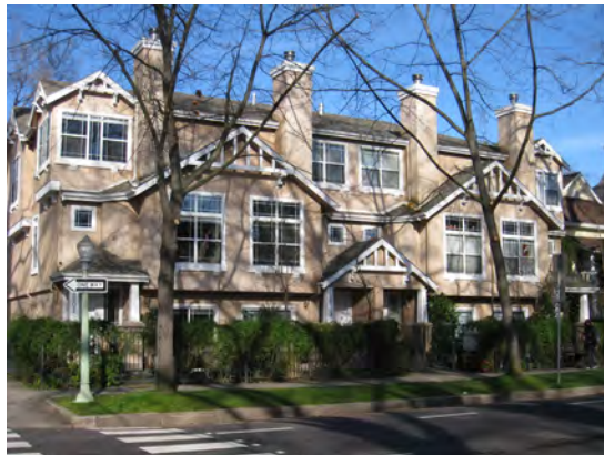
Units face the public street
