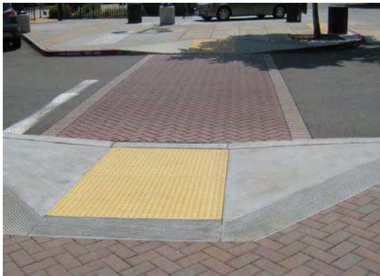
Ramp and warning strip
