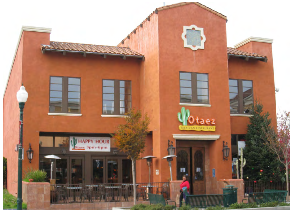
Varying cornices and rooflines
