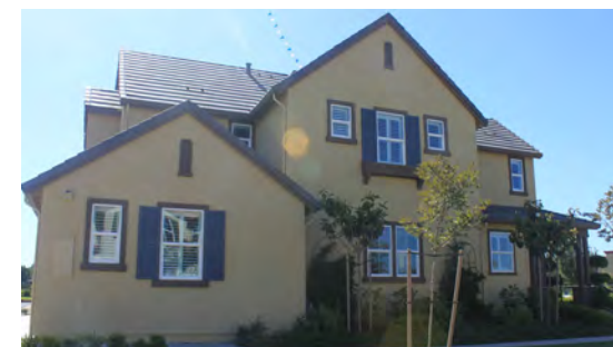
Enhanced window openings
