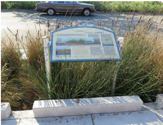
Landscaped stormwater planters
