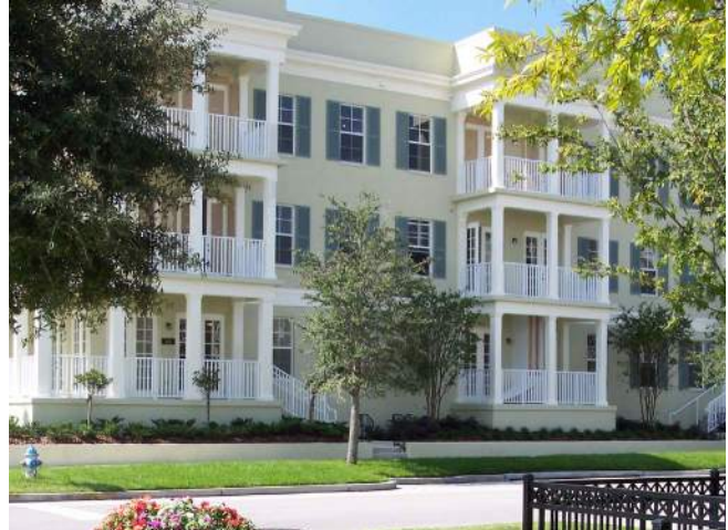
Multi-Level Courtyard Illustrative Photo
